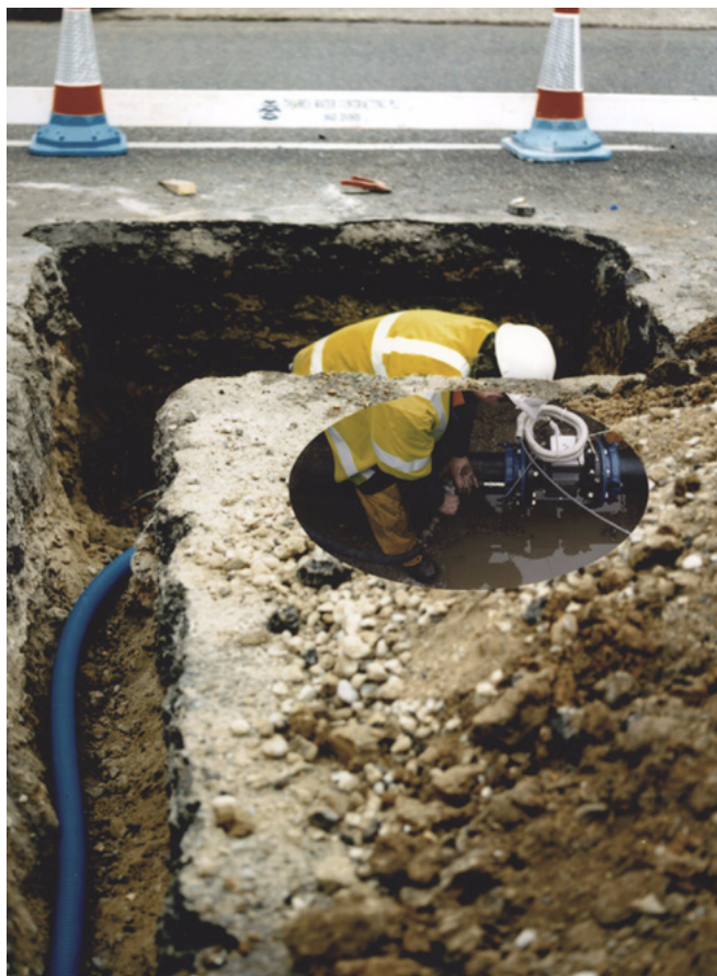
Underground Installation of MagMaster
